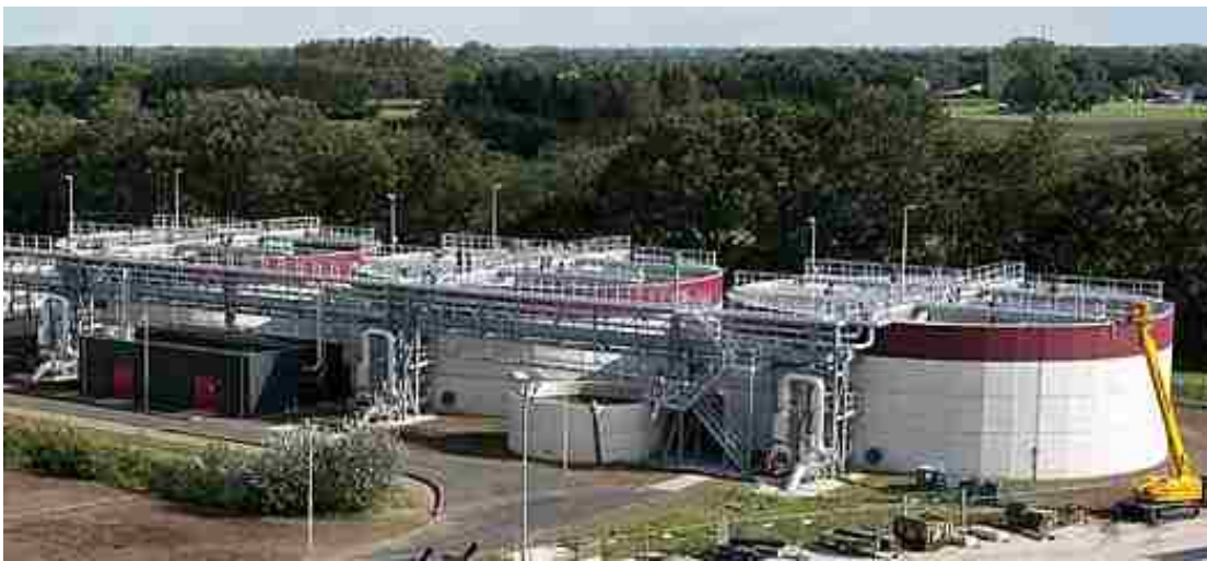
Figure 7-3. Aerial image of Nereda® Plant in Epe, The Netherlands. Reprinted with permission from the Netherlands Water Partnership. Copyright Netherlands Water Partnership. Retrieved from http://www.dutchwatersector.com/news-events/news/2704-official-commissioning-nereda-at-wwtp-epe-wonder-granule-keeps-its-promise.html
